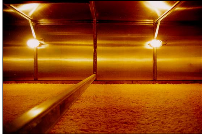
The inside of the drying tunnel
