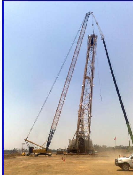
DRE12 Boom Point Sheave Upgrade
