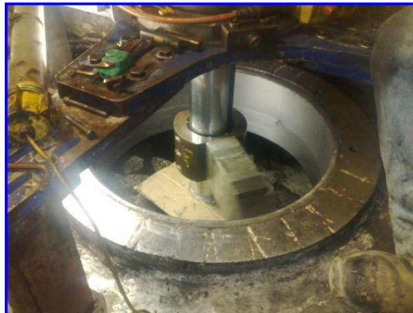
Line Boring of Lower Swing Bearing Cassette
