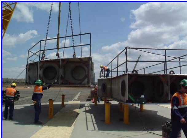
Marion 8050 Dragline Tub Erection
