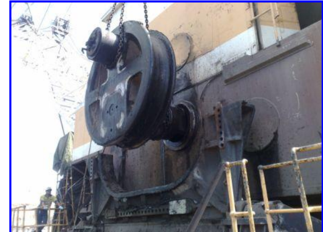
DRE21 LHS Propel Rebuild
