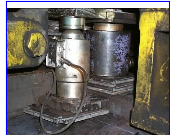
100T hydraulic jack and Load Cell under bogie
