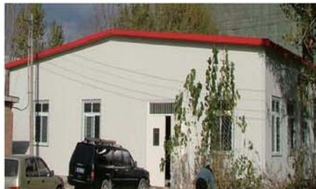
1. M style prefabricated house is a modular house with galvanized steel structure.
