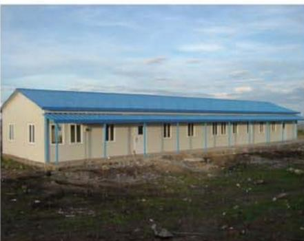
1. The house is made of light steel structure and rustproof color steel sandwich panel as wall and roof.
