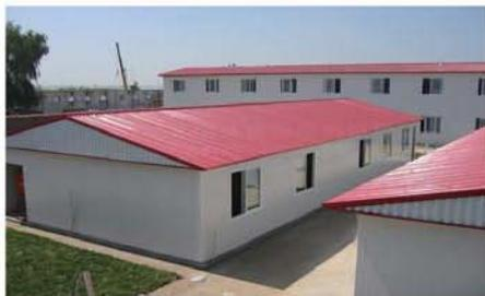
5. One 40HQ container can load about 160m<sup>2</sup> considering 75mm thickness panel for roof and wall;
