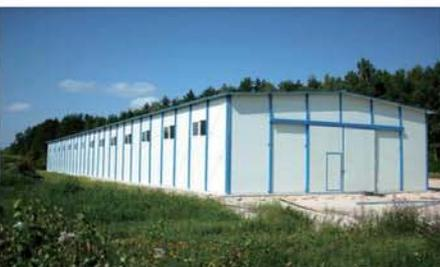
1. Rixin single storey or multi-storey is a modular house which width and length can be extended by adding number of 1820mm based on 3800mm.
