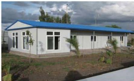
1. The house is made of light steel structure and rustproof color steel sandwich panel as wall and roof.
